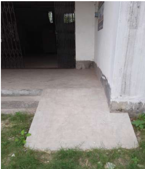
Ramp in the Annex building
