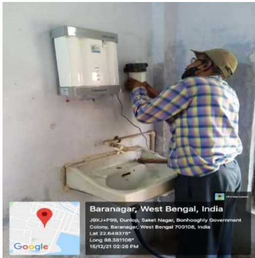
servicing of water purifier
