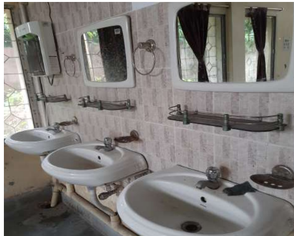
Taps with faucets
